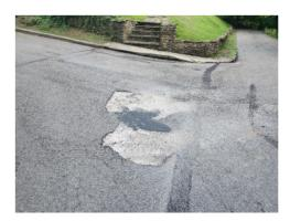
It is recommended that the Borough consider having Clovelly Road saw cut at the Briar Cliff burb line and approximately 5 feet above the damaged area. This section of the road should be removed, base repair should be performed. Then a new asphalt road section should be installed in this area.
